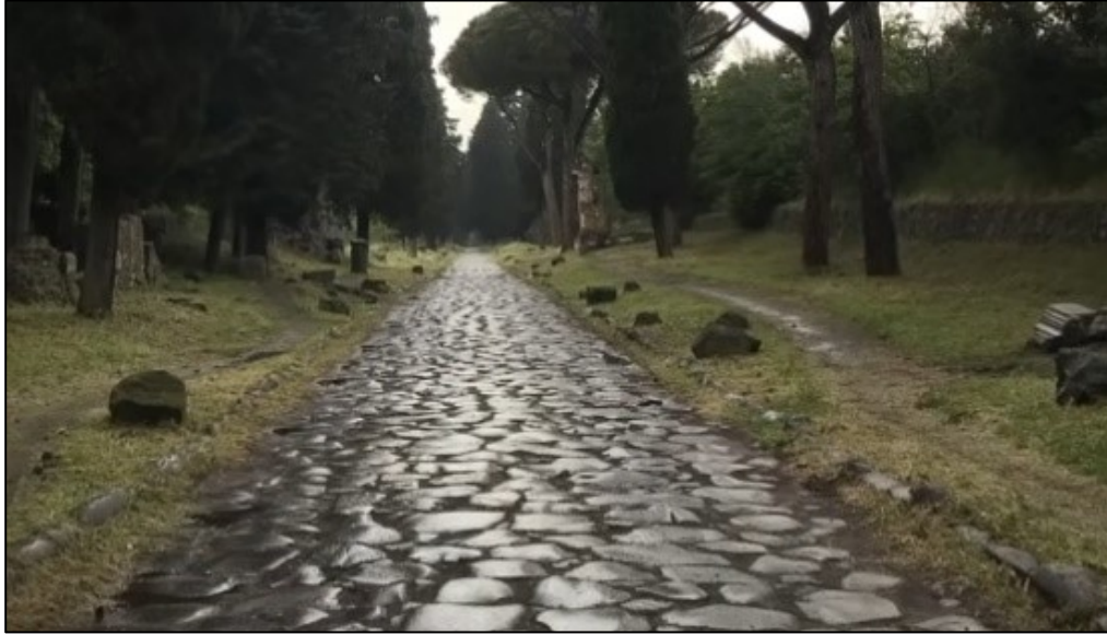
From YouTube Video: 'Were Roman Roads more Durable than Modern Highways' at 3:26 mins, illustrating the top rock layer of the Roman Roads polished by wear. https://www.youtube.com/watch?v=4egCVU3arVk
